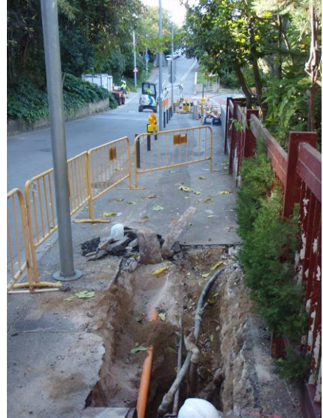
2. Vista general c. /Tres Pins.
